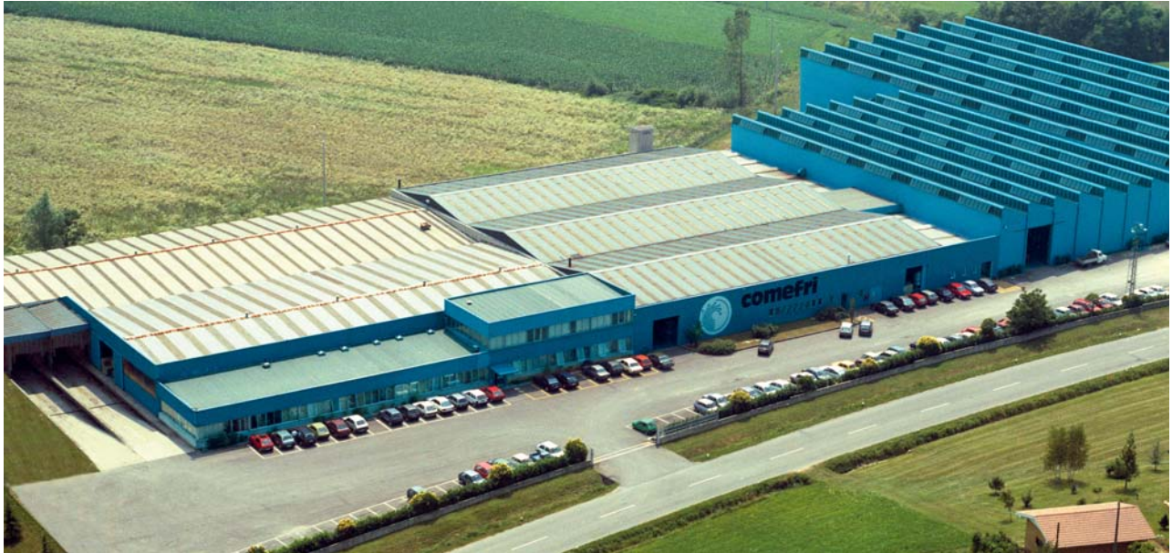
COMEFRI SpA factory at Magnano in Riviera (UD) - Italy with 156,000 sq.ft. manufacturing floor space, which produces radial fans for HVAC products.
